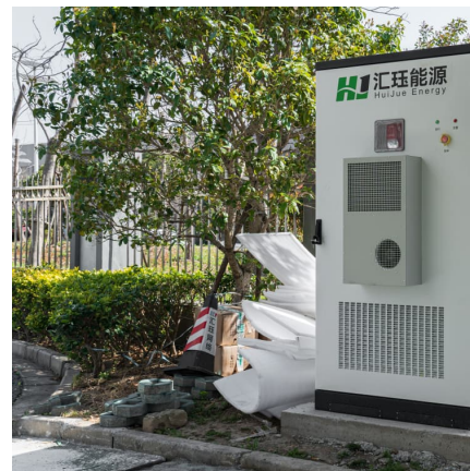
Energy Storage Cost and Performance Database
