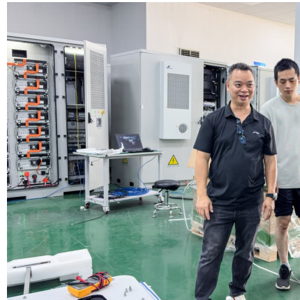
Battery energy storage power station logo image
