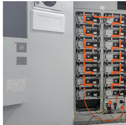
Energy storage welding column production
