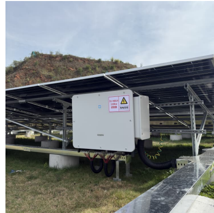
cairo henggang energy storage building
