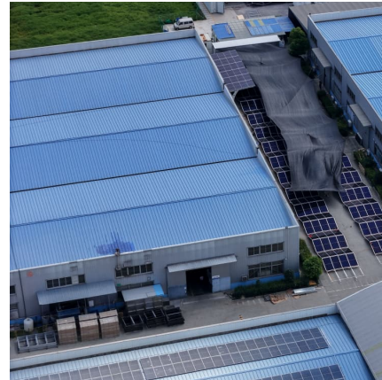
bangui energy storage power plant is in operation
