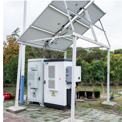
Utility-Scale PV , Electricity , 2023 , ATB , NREL
